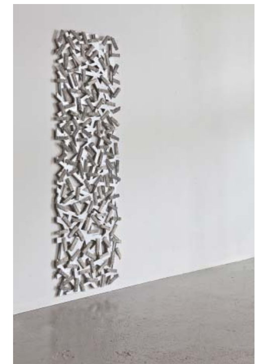
Ceramic Glazed Concrete, suspended curtain-wall constructionpanel 160-50-1-2 cm. Anja Margrethe Bache, Photos Ole Akhøj.
