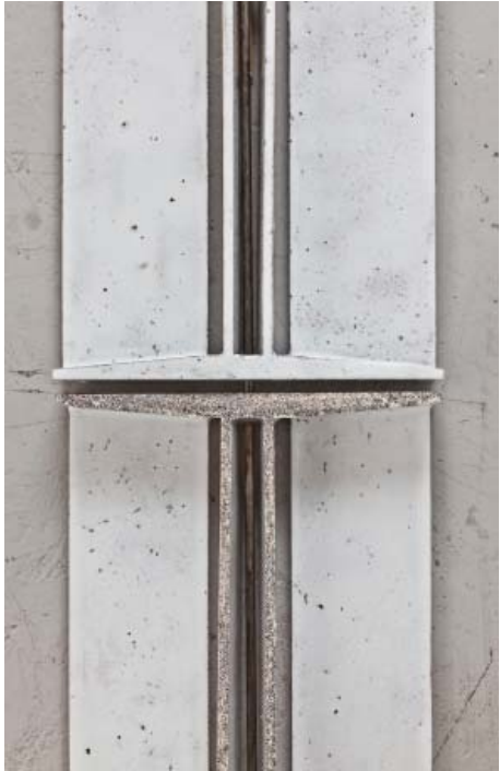
Ceramic Glazed Concrete, selfsupporting facing construction 160-50-1-3 cm. Anja Margrethe Bache, Photos Ole Akhøj.
