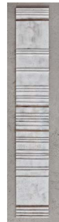
Ceramic Glazed Concrete and wood, suspended curtain-wall constructionpanel 160-50-1-2 cm. The wood is a part of the mounting system. Anja Margrethe Bache, Photos Ole Akhøj.
